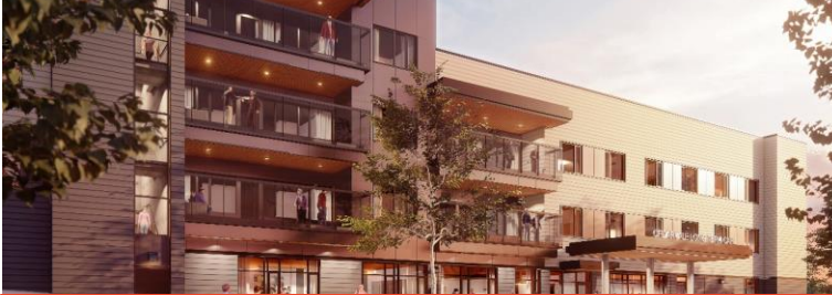
In Progress (Construction Start Q4 2024)
